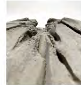
The flow of concrete illustrated in this photo is related to the reconnection of the broken building
