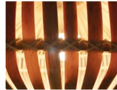
Knots tying together the sheets of bamboo
